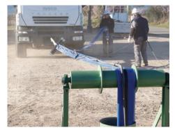
After initial installation, pump is lowered into well by use of a vehicle, with a single hose reaching depths up to 990 ft.
