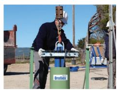
2. The install clamp is then used to lower the pump during initial installation.
