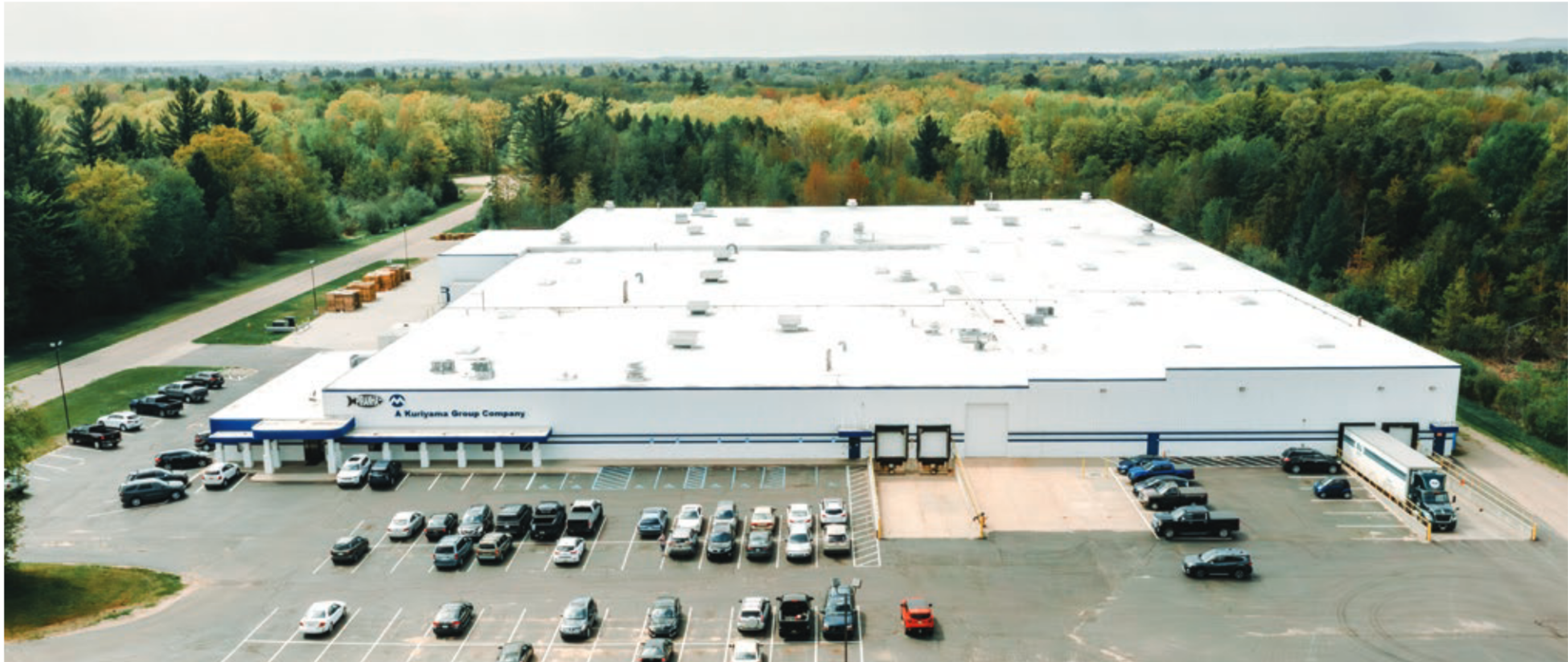
Piranhaflex Hoses are manufactured at Piranha's 178,000 sq. ft. facility in Cadillac, MI.
