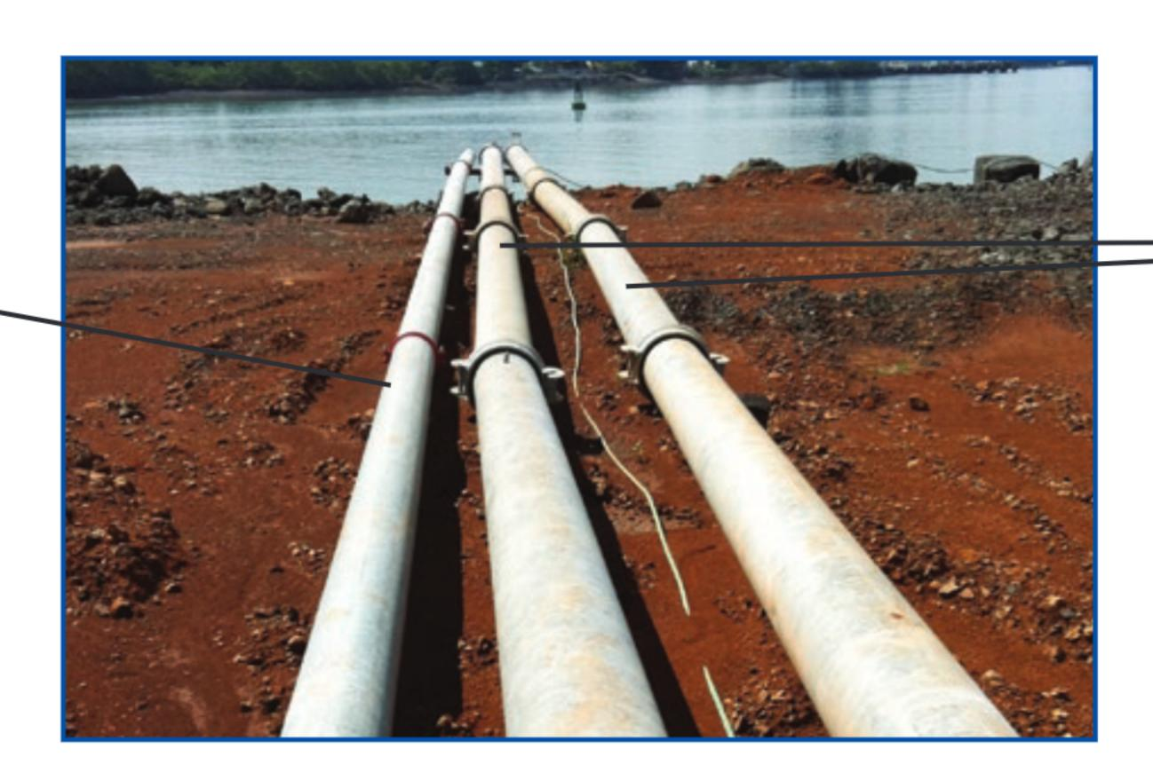
Sphere Lock couplings allow for angled/offset connections.
